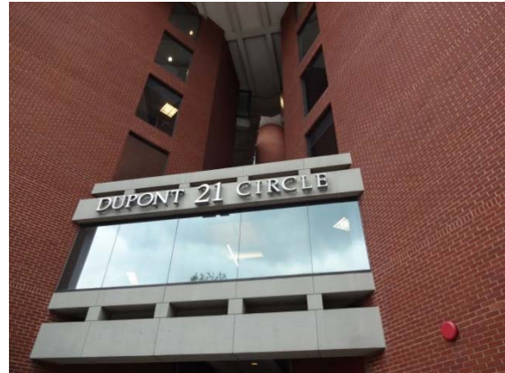
[ARLが入るビル]
